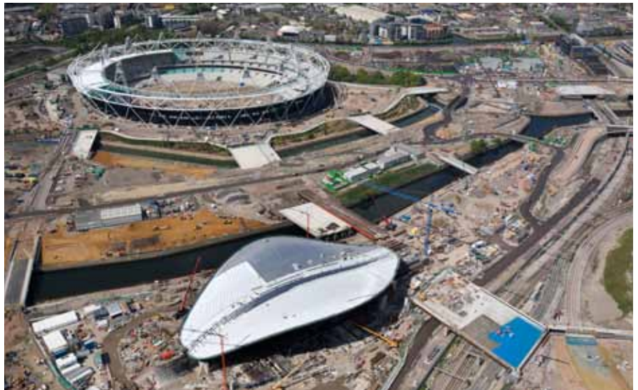
Aerial view of the Olympic Park during construction
