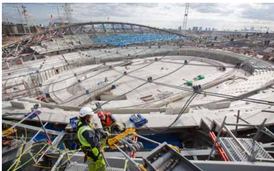
Workers lifting the Velodrome roof into place
